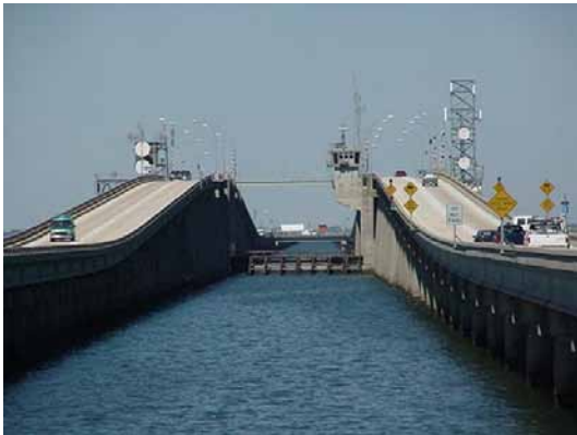
Figure 2—A new electrical system was needed to power drawbridge operation, cell phone towers, toll facilities, and a series of variable-message warning signs to be installed along the, oftentimes fog-enshrouded, causeway.
